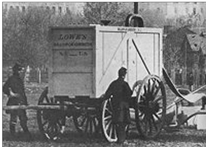
One of the logistical challenges faced by both sides was the availability of gas generators. Lowe solved this problem by developing a portable gas generator that provided greater deployment mobility. (Photo from the National Archives)
