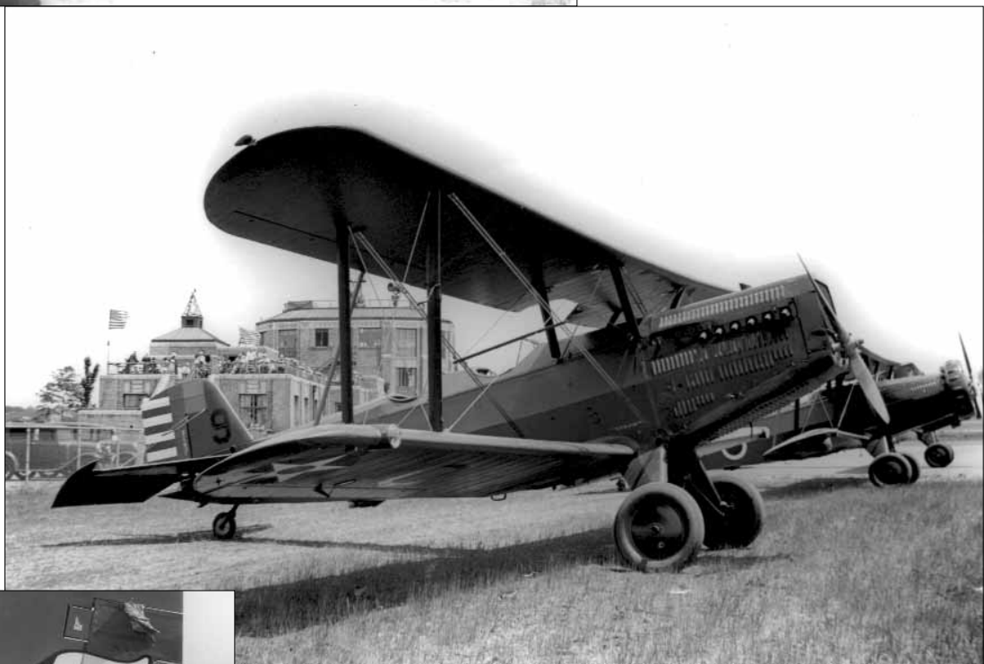
Right: Douglas BT-1 basic trainer converted from a O-2K Observation plane. Forty of 59 O-2Ks produced were reworked to the BT-1 configuration. This ship belongs to the 112th Squadron, Ohio National Guard. Akron Municipal Airport, Ohio, is the location. The Fourth of July 1933 is the occasion.
