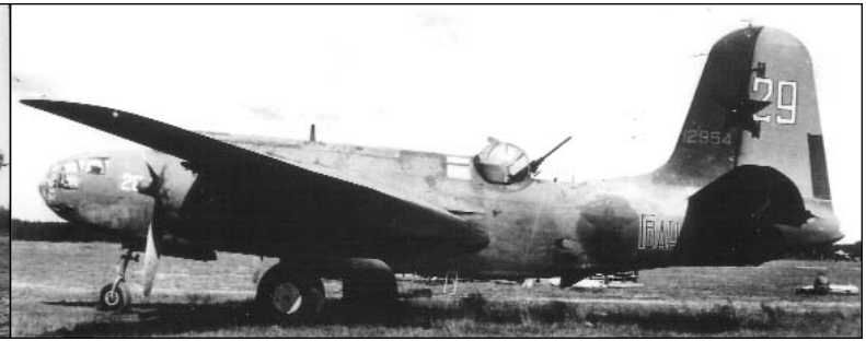
A-20B, 41-2954, nr 284/"29", inscribed "GVARDIYA," at NII VVS (Soviet Air Force Research Institute). Fitted with UBT 20 mm cannon in MY-3 dorsal turret. (Red Stars Vol. 4 provided by C-F Guest to author)
