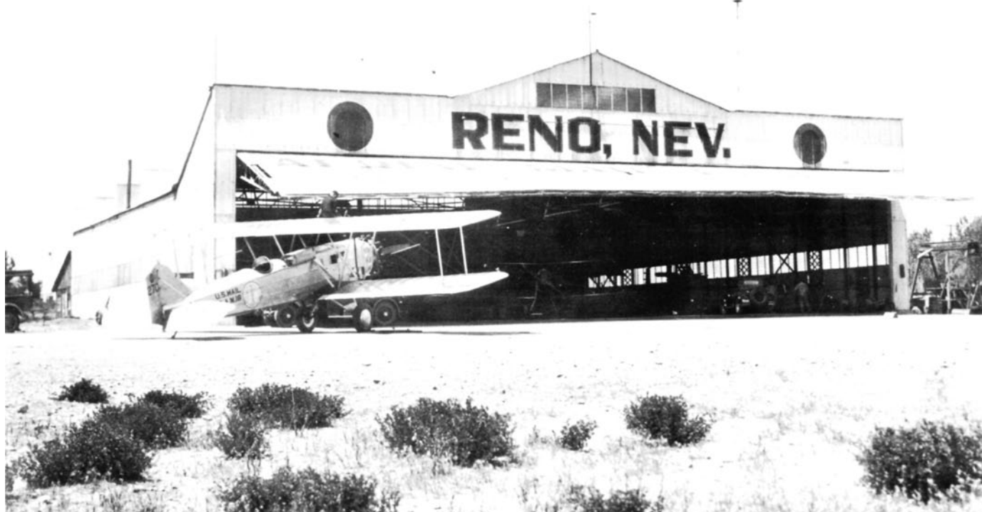
Above: Boeing 40A (registration number C 270) at United Air Lines Airport Reno, Nevada. Aft mail compartment is open and wing tank is being refueled. This aircraft originally went to Pratt & Whitney as an engine test bed. In it's later life it was converted to a two cockpit trainer. (Photo from United Airlines Archives)
