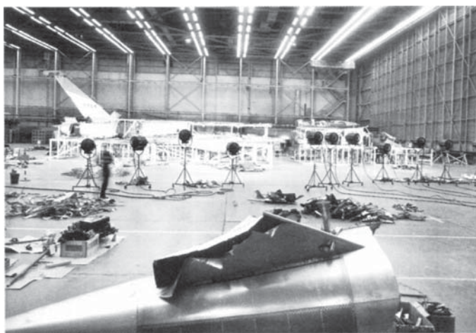
10: Remains of '5664 were transported by truck from Oklahoma back to Convair's Ft. Worth plant for partial reassembly in an attempt to ascertain the cause of the accident. In the foreground is the tail of the aircraft's MB-1 pod. (Photo from General Dynamics)
