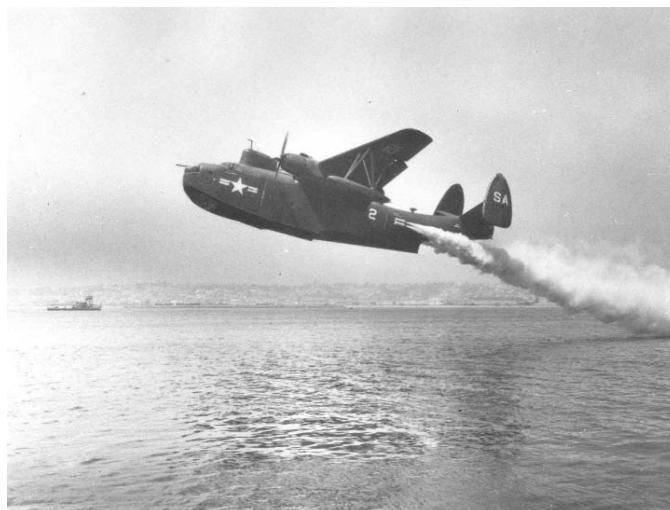
JATO helped to get this Martin PBM-5 off the water quickly. (Photo USN/Martin via Bruce Barth )
