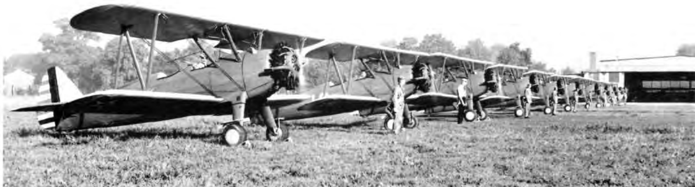
These 11 Stearman PT-13s are all prepared for flight at Parks Air College on May 28, 1940. The PT-13 was powered by a 215-hp Lycoming R-680-5 engine.
