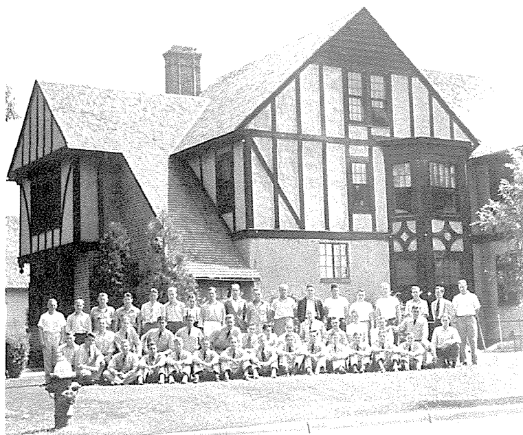
Classes 40-A (18) and 40-B (28) in front of the Cadet Barracks (converted frat house) across the street from Nebraska Wesleyan College, 5007 Huntington Avenue, Lincoln, Nebraska, 1939. (Schirmer Collection)
