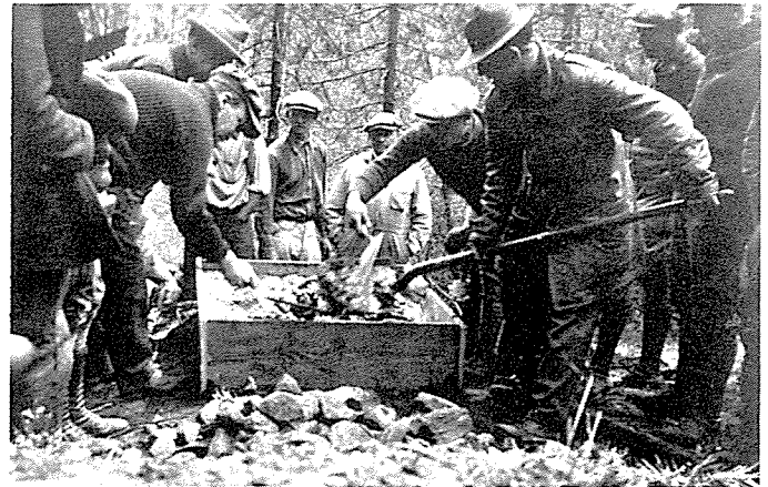
After policing the area, the Rockwell Field men mixed concrete for the monument. (Frank Curry)
