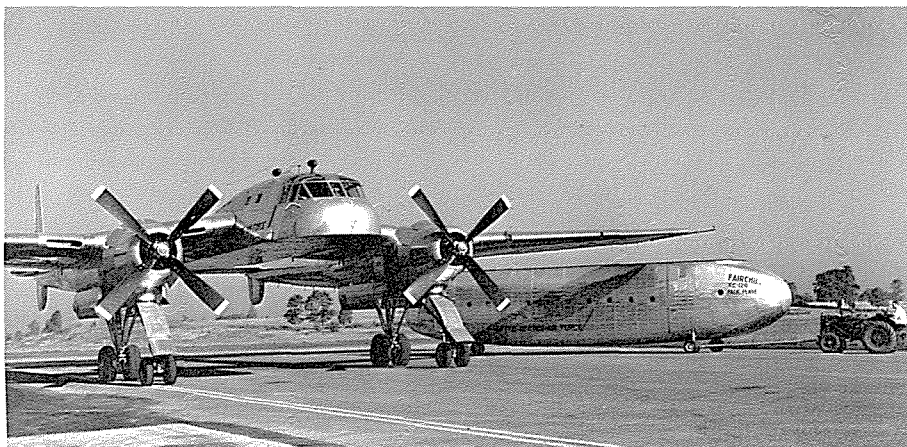
Towing the cargo pod clear of the XC-120.
