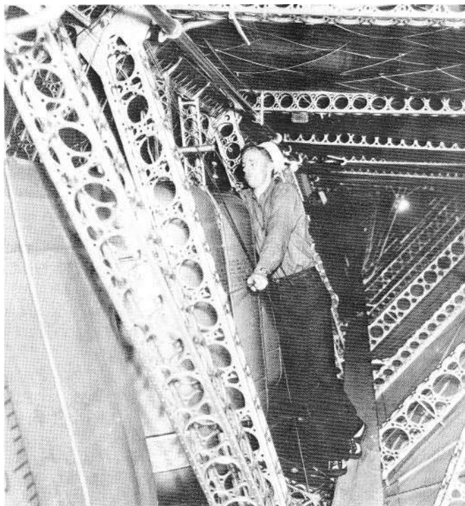
Crew member inspects fuel system of USS Akron. (National Archives Photo No. 80G-462606)
