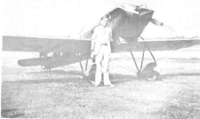
Jimmy Wedell standing in front of his We-Will prior to the 1930 National Air Races in Chicago. Note the chin radiator that has replaced the wing radiators. Also the wheel pants which was the beginning of the wheel covering that marked the Wedell-Williams racers.
