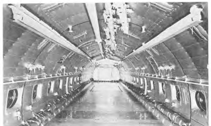
A C-47's interior arranged for heavy cargo. Gun port corks attached to strings can be seen in the windows. Litters can be seen stored below the windows and the overhead tracks are for cargo tiedown and off-loading. (Harry Gann DAC)
