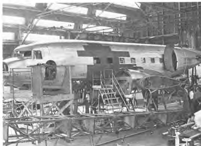
Production line converting DC-3 into Super DC-3.
