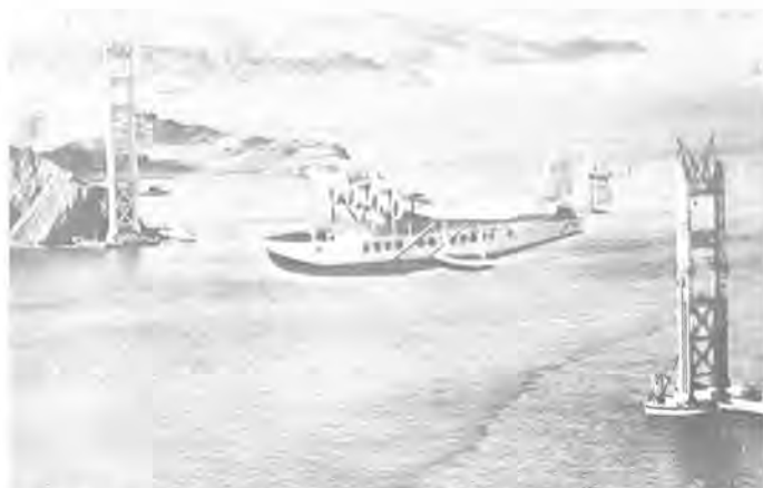
The S-42 trans-Pacific survey plane, Pan American Clipper , departing San Francisco on the first leg of the proposed Pacific airway, April 16, 1935. Note that the cables of the Golden Gate Bridge have not yet been hung at this point. Survey crew: Capt. Edwin C. Musick, First Officer R.O.D. Sullivan, Navigator Fred J. Noonan, Junior Flight Officer Harry R. Canaday, Flight Engineer Victor Wright, Radio Officer Wilson T. Jarboe, Jr. (Pan Am File Photo via Dick Kruse)
