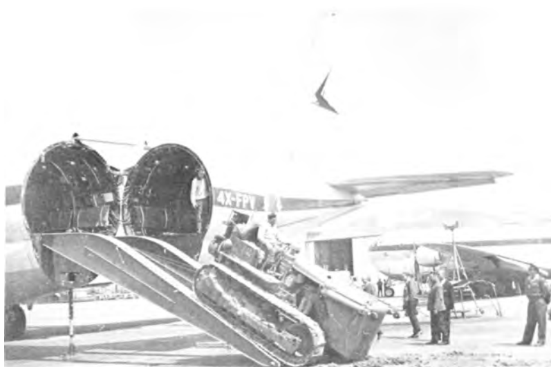
A close view of 4X-FPV's swing-tail conversion with a tractor being unloaded. This modification was the first and only done on the B-377. Parked next to it is aircraft No. 15 (4X-FPW), the second swing-tail conversion. (Author's Collection)
