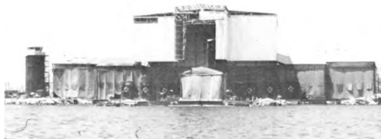
Harold Tegart designed a permanent cruciform hangar for the Flying Boat. Aluminum siding replaced the canvas panels. (Elmar Baxter Photo)
