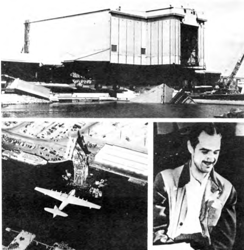
In 1980 the hangar doors had not been raised in 20 years. Demolition crew cut the doors off in order to remove the flying boat. The Navy's crane, Herman the German, moved the Flying Boat out of its hangar in early 1981. Howard Hughes at work. (Port of Long Beach Photos)
