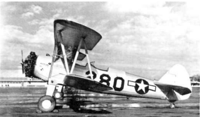
Stearman PT-13D used the Lycoming R-680 engine. Some pilots preferred the somewhat smoother Lycoming to the Continental. (Bob Markow Photo)
