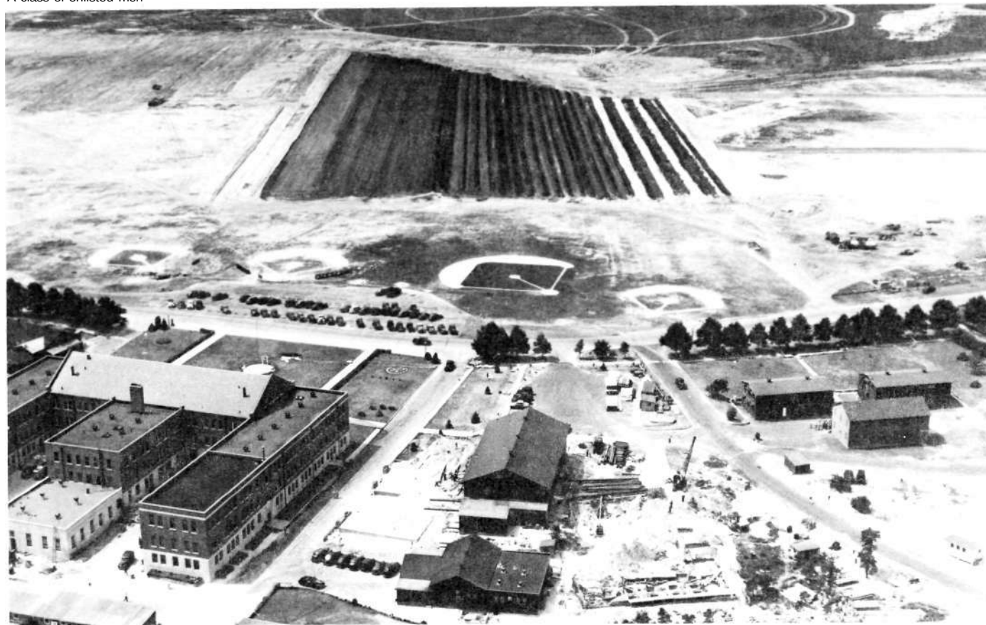
The paving of Mat 1
