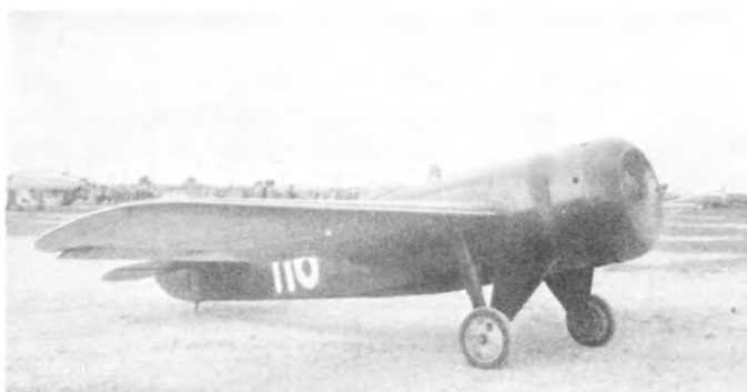
Two photos of the Cessna GC-2. It was the same as the GC-1 but powered by a Warner Scarab engine.
