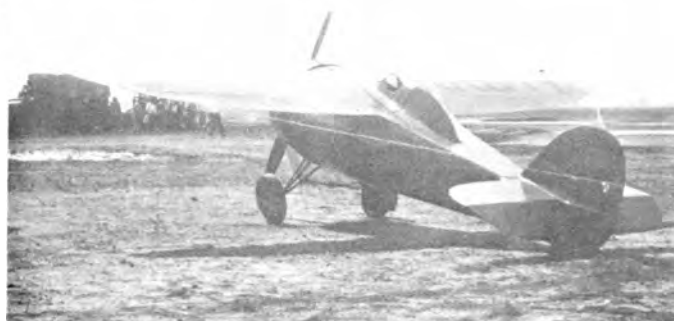
Side and three-quarters rear view of CR-3 after Livingston's modifications of lower canopy with open headroom at top and wheel enclosure panel added to gear. Livingston's license number was 1427. He used 14 for the race number on his Monocoupe and 27 on the Cessna.
