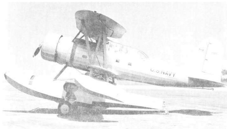
Left side view of the XO2D-1, April 19, 1934. The left water rudder can be seen flush mounted between round access plates at the rear of the main float sides. (MDC via Bob Williams)
