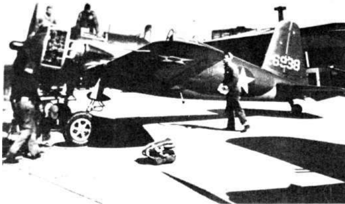
P-66 in defensive pursuit service. 14th P.G., Oakland, Ca. NAS, Feb. 1942. Note that even in pristine stateside conditions, the lower wheel cover is removed. (S.C. Timson)
