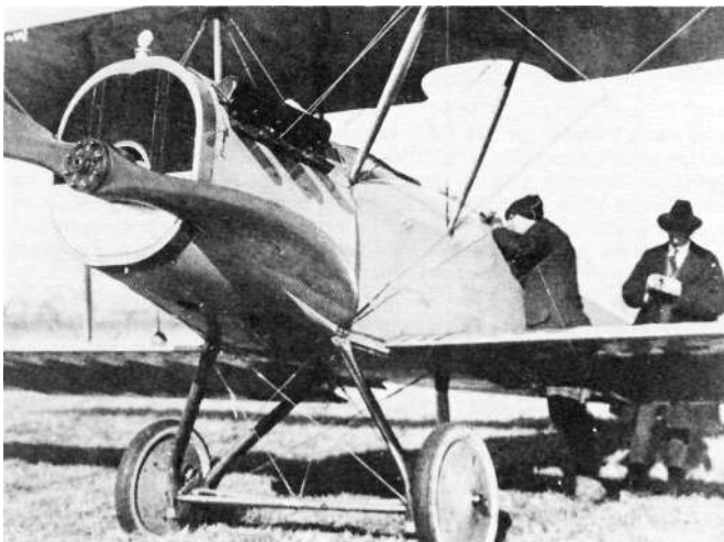
Wright-Martin V designed by Chance Vought for the aircraft company he worked for briefly as chief aeronautical executive engineer. The company was formed during World War I by merging the Wright Aircraft Company, the Glenn L. Martin and the Simplex Automobile Co. The Wright-Martin V was the first American plane to have the European Hispano-Suiza 150-hp engine so successful during the war. The company devoted so much of its energy to developing the engine it did not push the plane design, only one of which was built and first flew in 1915. (Photo from Vought Albums)
