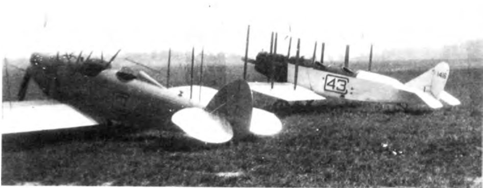
Clipped-wing Standard with OX-5 or OXX-6 and nose radiator. Note that fuselage deck drops more abruptly than N-B types, just in front of the fin. This could possibly have been a Robertson, but with so many variations of Standards, who knows?
