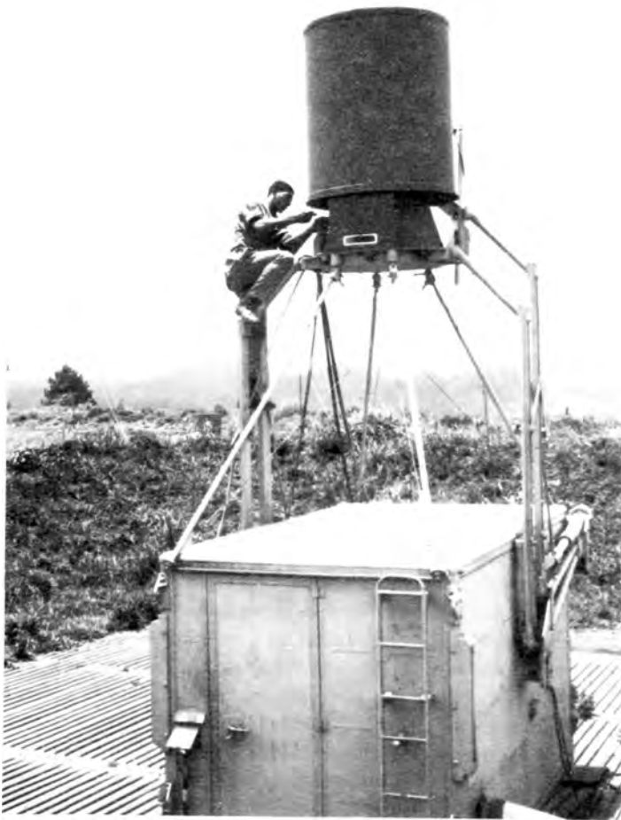
U.S. Air Force Sgt. Evans Long, Jr., of the 1882nd Communications Squadron, adjusts an AN/TRN-6 TACAN at Cam Ly Airstrip, South Vietnam. May 1969. (Official U.S. Air Force Photo)
