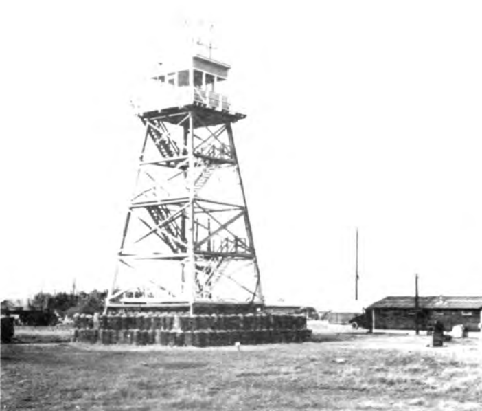
Control tower, Kunsan Air Base, Korea. Dec. 1951. (Official U.S. Air Force Photo)
