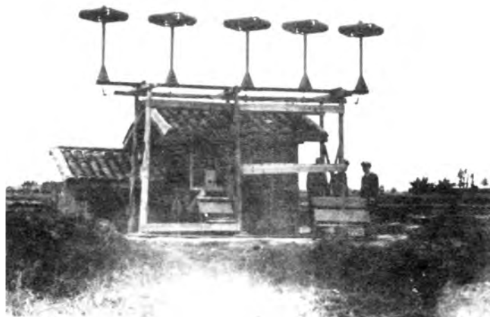
SCS-51 instrument landing system installation of the 4th Army Airways Communications System Wing at Kwanghan, China, Nov. 1944. (Official U.S. Air Force Photo)
