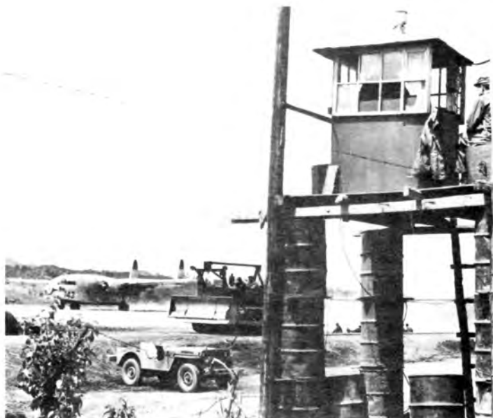
An AACS operator in this crudely constructed but serviceable control tower has cleared a U.S. Far East Air Forces C-119 Flying Boxcar to land at an advanced Korean airstrip. U.S. Army engineers continue with their construction work as the transport lands. June 1951. (Official U.S. Air Force Photo)
