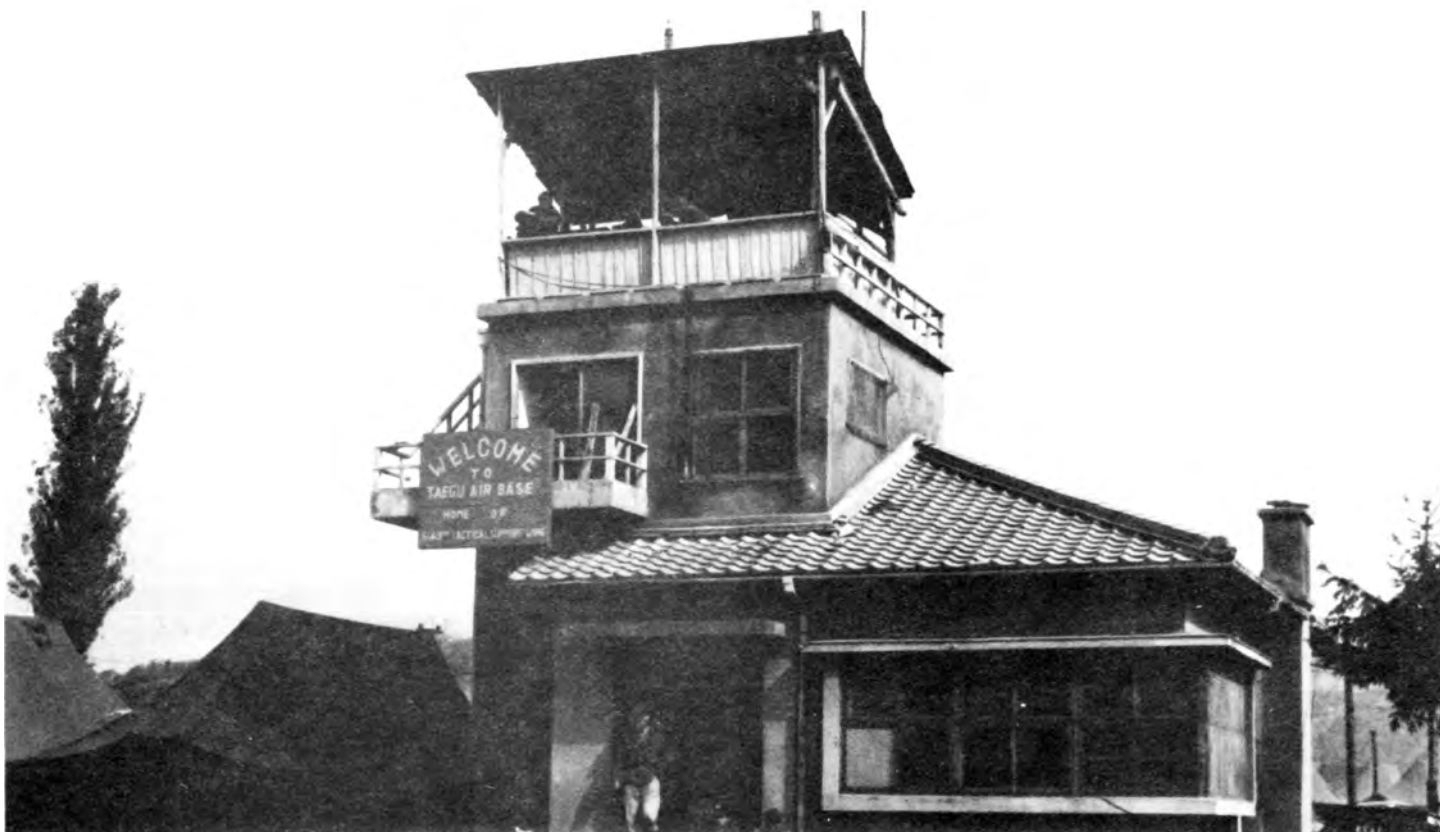
Typical of the Ingenuity of the U.S. Air Force in Korea was the addition of the perch atop an old Korean building at Taegu, in order to provide an "open-air" control tower for operations of the fighter strip located there. Oct. 1950. (Official U.S. Air Force Photo)
