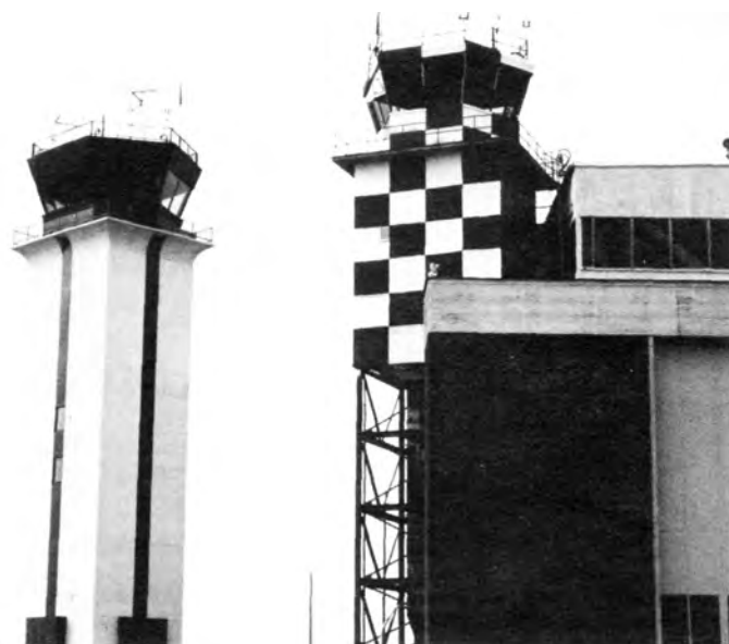
Griffiss AFB, N.Y.—The old red and white tower is being dismantled, and the new white tower will be operating in its place. August 1980. (U.S. Air Force Photo by 2Lt. Jan Wood)
