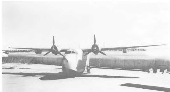
The Model 31 at San Diego, May 1939, showing mooring hatch in nose and original Hamilton Standard 15% \pi -diameter props.
