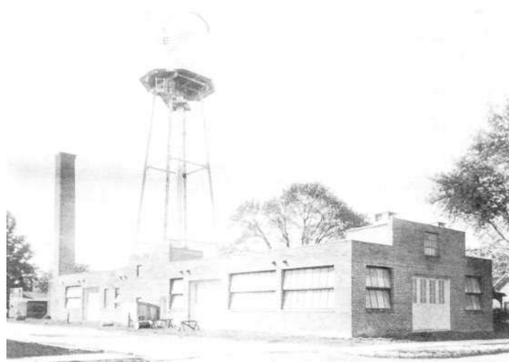
Exterior view of the $40,000 N-B dope building. The special windows on the left are hinged at the top of each frame. If dope fumes inside the building exploded, the entire window frame could pivot outwards to relieve the pressure. The windows would then fall back into their normal position. The chimney and heating plant for the entire N-B complex are behind the dope building. (C. Buckner, Jr.)
