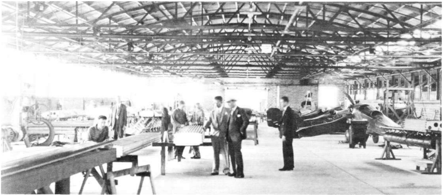
West end of Sec. No. 3 (300'x75') showing clear span roof construction and ventilation sash. A portion of the wing shop was moved to this building. The NB-3 on the right facing away is D/Comm. No. 2834 (No. 12) with a LeBlond engine. The first NB-3 facing the right wall is D/Comm. No. 358 (No. 4) with a Superior Radial engine. The men are unidentified. (C. Buckner, Jr.)
