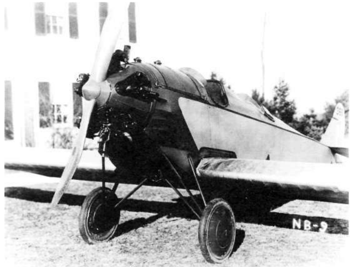
NB-3 D/Comm. No. 356 (No. 2) showing the early nose configuration as designed by Barling. Note the location of the oil and fuel tanks immediately behind the engine. This led to some instability problems. (R.B. Nicholas)
