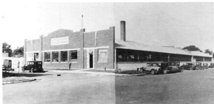
A composite photograph showing N-B Buildings No. 1 (to the left front) and No. 2 (to the right rear extending beyond the firewall). The gate and remaining lattice fence at the far left are a remainder of the old Wingfield Hitchyard. The light-colored area immediately above the fence is the roof of those sheds. (C. Buckner, Jr.)
