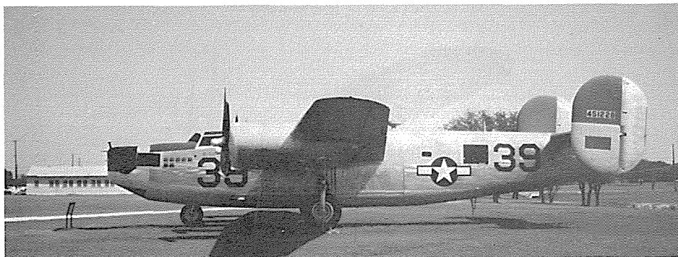
This C-109 look-alike is a B-24M-20-FO which was used in an icing research project after WWII. While its nose fairing does not have the typical C-109 profile, its tail fairing is identical and all turrets were removed. (Author)
