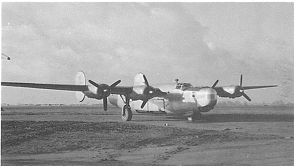
These two photos of a IX Troop Carrier Command C-109 (B-24J-15-FO) were taken in England during December 1944. Note the 90-degree arc on the profile of upper portion of the nose fairing. This curvature is a recognition feature for production C-109s. The bottom portions of the four bomb bay tanks are clearly visible in the lower photo. The standard C-109 had two Automatic Direction Finder "football" antennas on the fuselage top while most B-24s had only one. (USAF)
