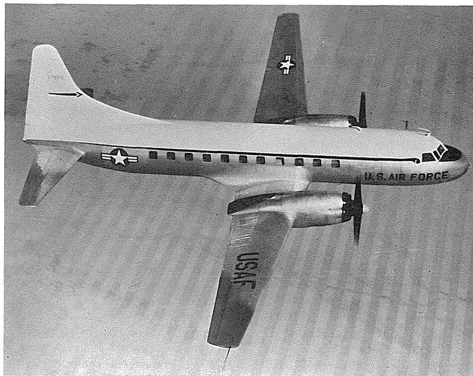
YC-131C 53-7886 with test instrumentation on right wingtip. The YC-131Cs featured a 40-inch extension to horizontal stabilizer and a 12-inch tail extension. (Air Force courtesy of Robert F. Dorr)
