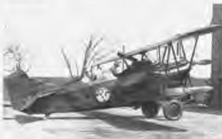
Two views of the Curtiss Falcon owned by Wright Aeronautical for flight testing the G.E. turbo-supercharger. Photo taken ca. 1933-1937.
