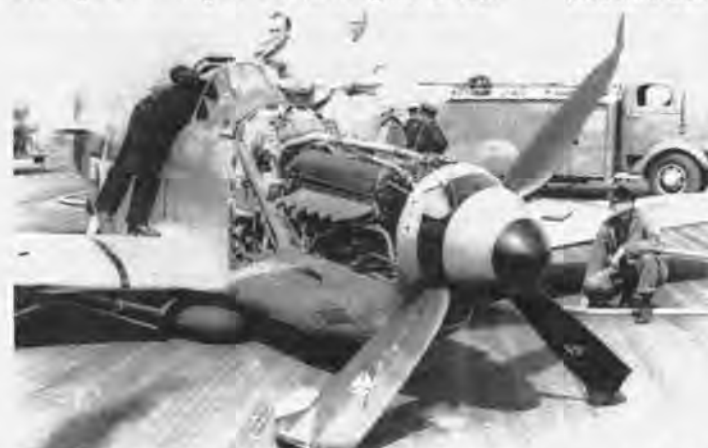
P-51H, 44-64183, was written off on July 19, 1945. It appears that the pilot attempted to recycle the landing gear from a mid-position in its travel. The end result was a pair of crushed wheel well covers, jammed landing gear, and one less P-51H. (NAA courtesy of Gene Boswell)
