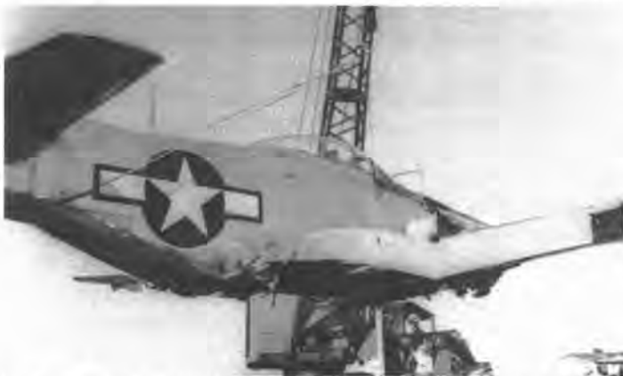
On Feb. 6, 1945, Bob Chilton's birthday, the first P-51H, 44-64160, suffered a propeller failure. Chilton force landed near the Hollywood Race Track, touching down just short of a ditch, shedding the radiator and doghouse on the bank, followed by the prop. The airplane was a write-off, but was used as an instructional airframe for two years before being scrapped. (NAA courtesy of Gene Boswell)
