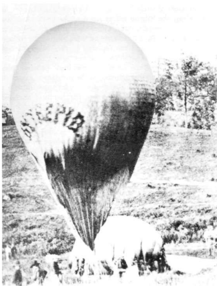
Lowe's portable hydrogen gas generators in action. Lowe can be seen at the far right of the picture testing the expanding envelope. (Smithsonian Institution)
