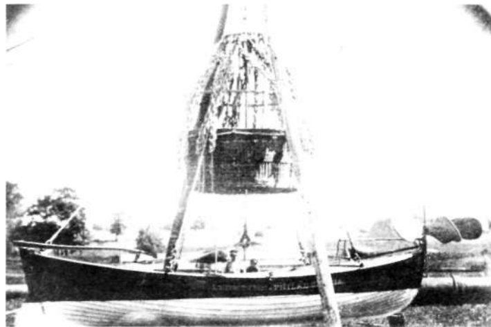
The 30-foot lifeboat Leontine shown slung beneath the basket of the City of New York in a test suspension from a gin pole. The six-bladed horizontal propeller mounted on the prow was to have been driven by a four-horsepower steam engine, but is shown in the photo to be only hand-operated. With it Lowe hoped to control the balloon's altitude, thus eliminating the conventional method of discarded vitally important ballast—the very life blood of any balloon. Whatever prompted this idea—facetiousness, publicity or ignorance—is not known, but quite obviously it would have been utterly useless. (Smithsonian Institution)
