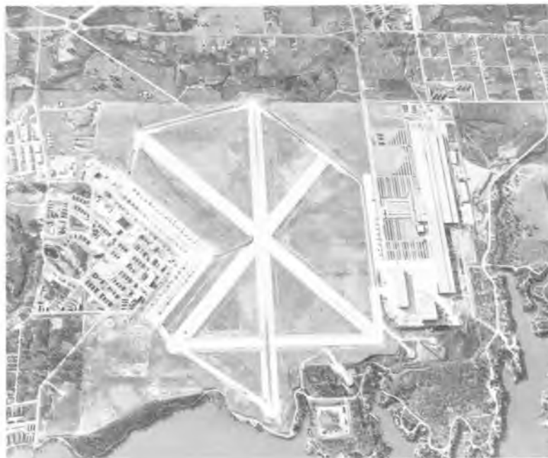
Aerial view of Fort Worth Army Air Field (left) and center runway shared with Convair's near mile-long aircraft factory. Lake Worth forms northern border at bottom of photo, 1944. (General Dynamics, Fort Worth)
