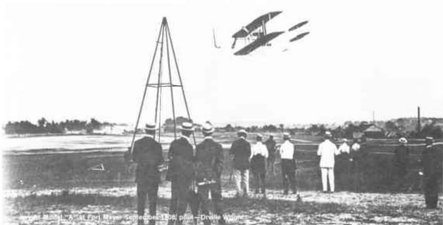
Wright Biplane Model "B"; 30-hp Wright—4, Span 39', Length 26'
