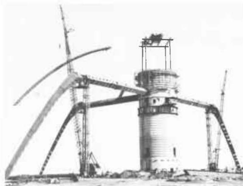
The new air terminal at Los Angeles International Airport was built in the late 1950s. Here the parabolic arch-shaped Theme Building, to house a restaurant and observation deck, is being constructed. (Los Angeles Department of Airports)
