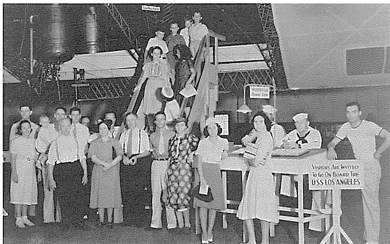
Visitors pause for the photographer beneath the decommissioned LOS ANGELES in Hangar One. A section of the outer cover has been removed, some of the airship's equipment has been labeled, and a platform access provided to the keel. Never before had the casual Lakehurst visitor been permitted onto the "catwalk" of a Navy rigid. Note the lacing cord for the adjacent panels of outer fabric. This photograph, dated 19 July 1939, is published here for the first time. (U.S. Navy photo courtesy of the late C.M. Ruth)
