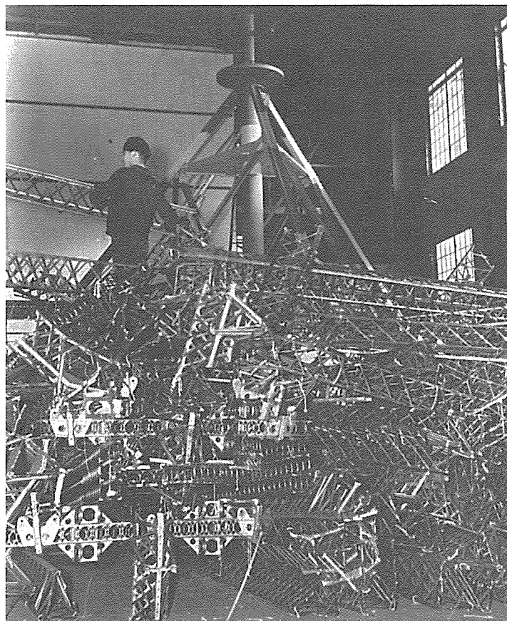
Visitors pause for the photographer beneath the decommissioned LOS ANGELES in Hangar One. A section of the outer cover has been removed, some of the airship's equipment has been labeled, and a platform access provided to the keel. Never before had the casual Lakehurst visitor been permitted onto the "catwalk" of a Navy rigid. Note the lacing cord for the adjacent panels of outer fabric. This photograph, dated 19 July 1939, is published here for the first time. (U.S. Navy photo courtesy of the late C.M. Ruth)
