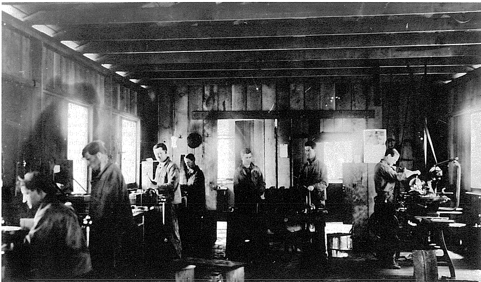
The engine repair shop and mechanic's school at the Signal Corps Aviation School, North Island, San Diego, California, in about 1915. Excellent work
