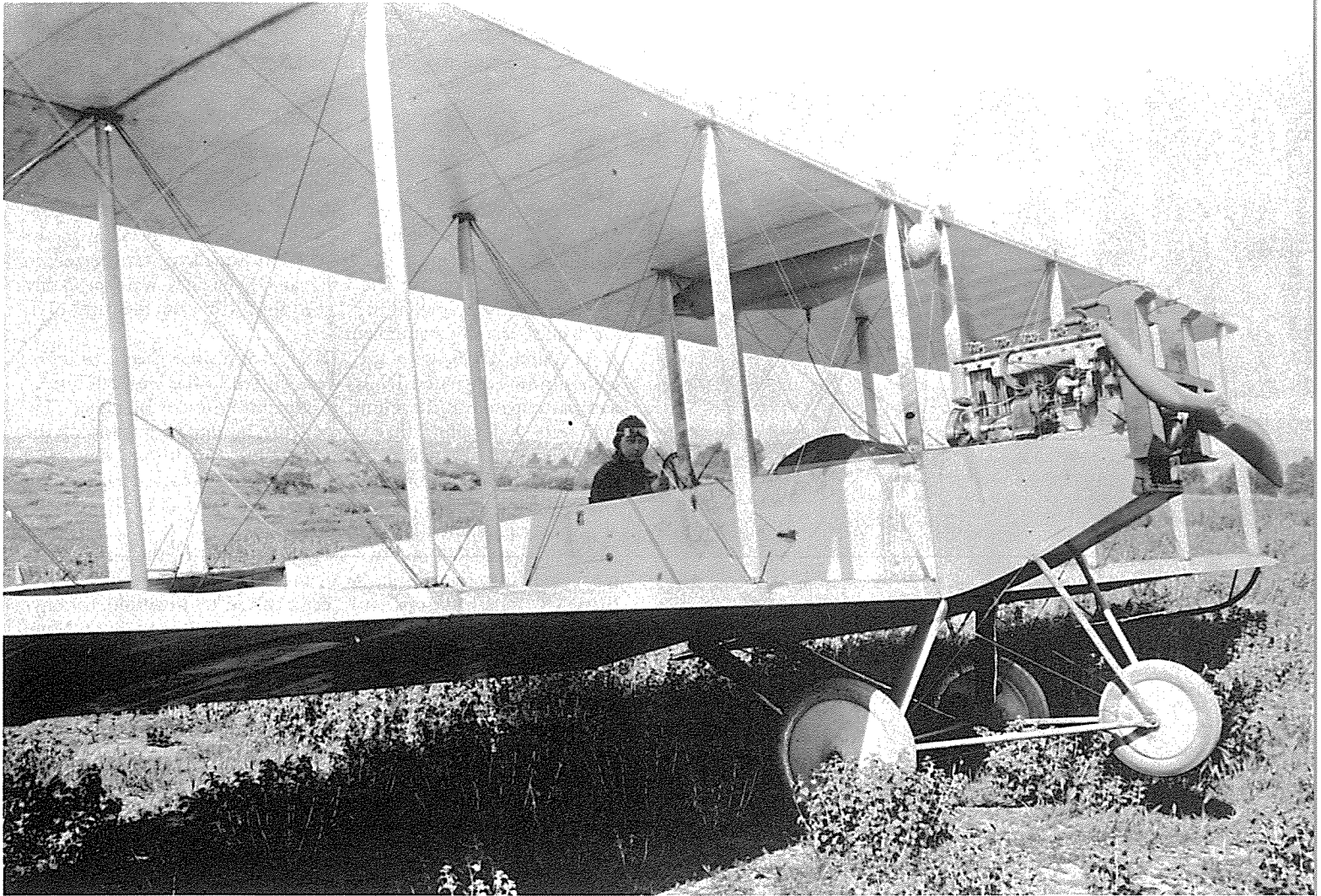
Only one 6-cylinder Curtiss S engine was purchased by the Army. This 60-h.p. unit was installed in the Curtiss Tractor trainer of 1915 shown above which was rejected by the Army. The powerplant was then used in
