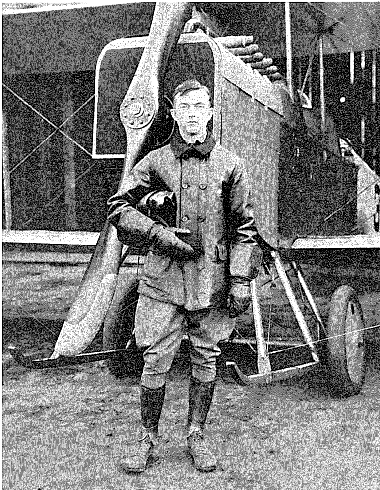
Curtiss N Number 35 was modified to use the odd Beardmore 90-h.p. engine originally installed in the Wright F catastrophe. Built in England, this excellent 6-cylinder engine is barely visible, though the light-colored upper cowl identifies one of the alterations made to accommodate the unit. Lt. Clinton W. Russell is the pilot. (National Archives)
