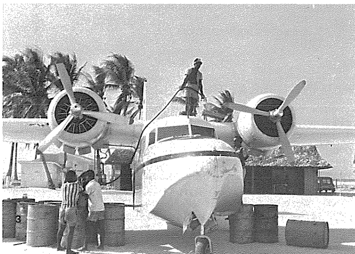
6. Fuller Brush Company's N2943 (J6) is shown in a 1946 photo. Note the sawhorse used prior to installation of the "squat strut." Leading edge slot is also evident in photo. Propeller warning stripe is unusual on Mallards. Peter M. Bowers
