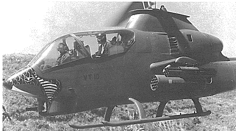
(Below) Marine Corps pilot transition training in AH-1G 815046 at Hunter Army Airfield, Fort Stewart, Georgia. Mid 1969. The large numbers and light-colored areas on the forward fuselage are day-glo orange with the standard yellow tail rotor warning strips around the tail boom. USMC A419214
