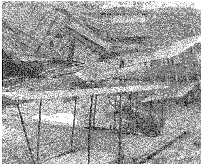
(Below) Hangars damaged by wind storm, 1917. Planes in hangars were relatively undamaged.
