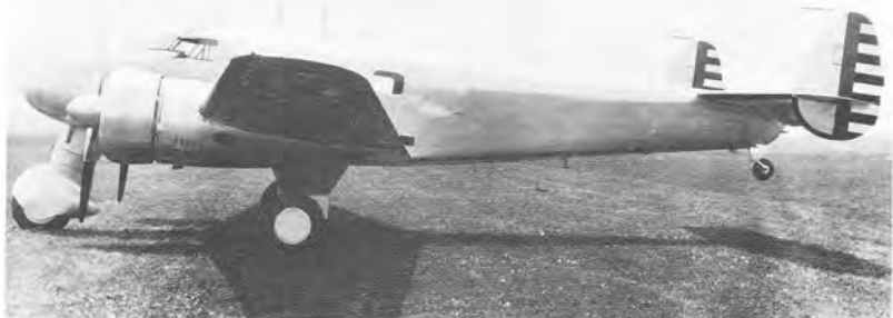
(Above) Sprouting an extra whip antenna, the C-40B was a radio test airplane during the pre-war years, and was converted to a standard C040A later. (National Archives 18-WP-64443)
