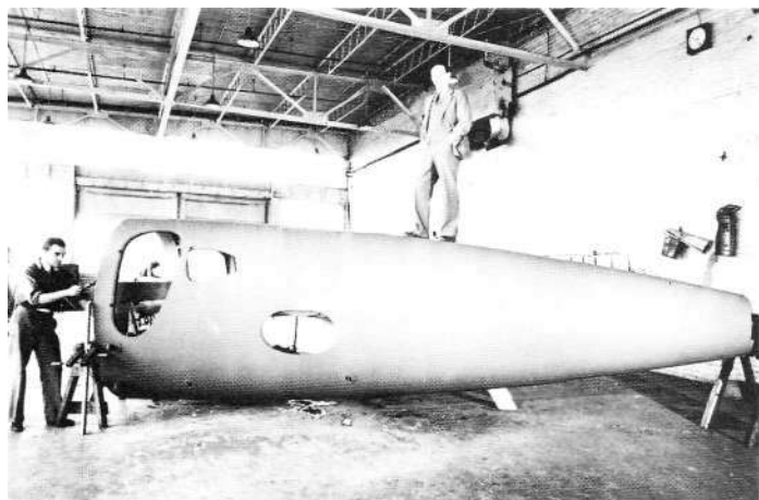
Above, the fuselage shell made by the Haskellite Company by a process later to be called "Duromold Process." Below, left and right side views of the Ranger V770 engine installation. Opposite page, the F46A over Hagerstown after gaining the NC registration. (Photos — Fairchild)
