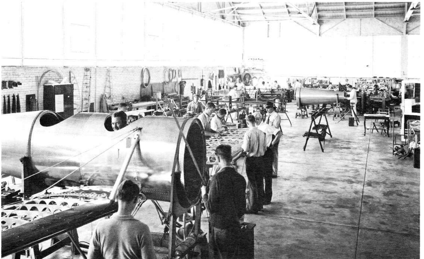
These two views of the assembly and fabrication areas of the Ryan School of Aeronautics were made in latter 1935 as production got going for the sport-plane market. 27 men were producing one S-T every second week, but of course later, as pre-war military orders came the whole operation was done in new and larger facilities. (Photos— "Erickson 35-152-1 (Upper) and 35-119-2 (lower)"
