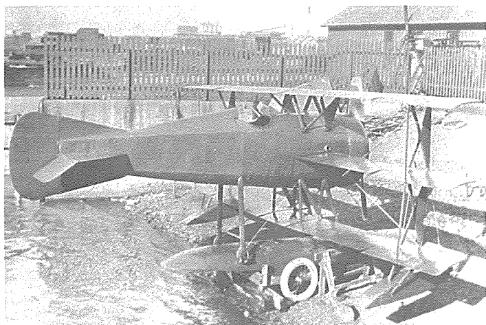
GS-1 - The Gnome Scout One - also called "The Door Knob Control", with shock absorbers in the pontoon struts. (NASM)
