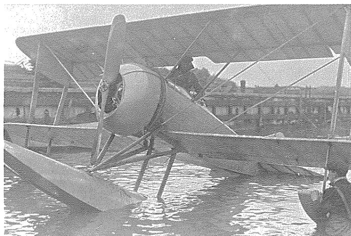
GS-2, called "The Swiss Cheese" by the shop crew because of the tailpost design with lightening holes. It sat on its tail in first test. (NASM)
