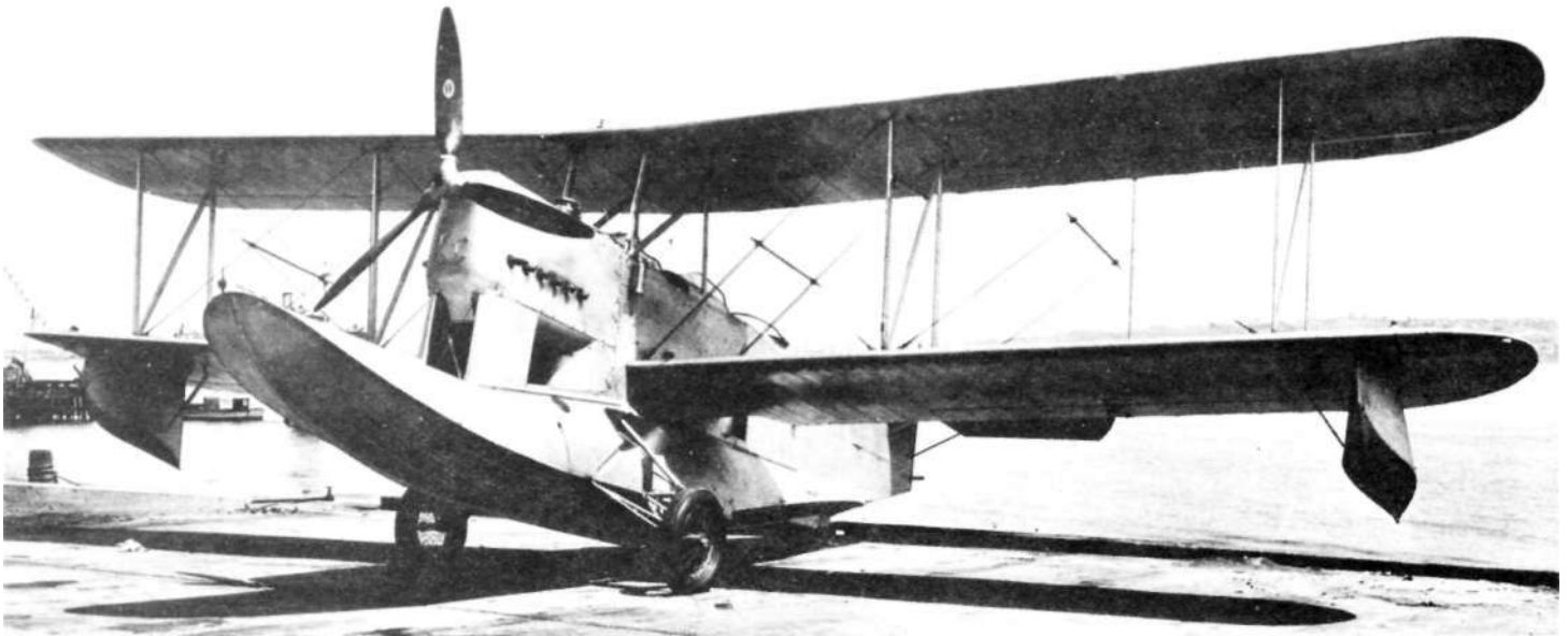
The Hamilton Standard propeller increased both weight and performance. (Nat'l Archives 80-G-3146, courtesy of Fred T. Donaldson)
