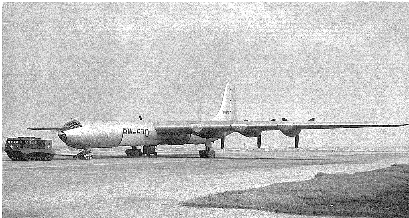
The XB-36 in mid-1950, being towed out for taxi trials on the new track type landing gear past Carswell AFB in background, showing eleven B-36's on the line. Sliding doors on bomb bay No. 1 are open. These were later changed to snap-open, two-section type in production. (Photo - Convair 10-4581)
