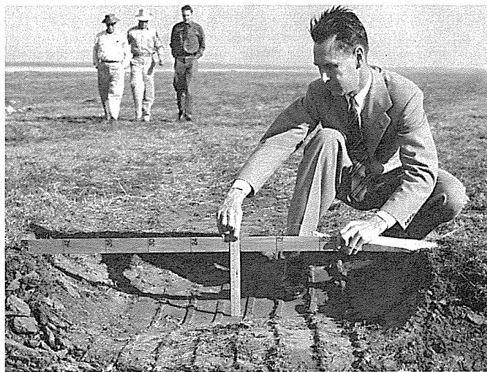
The size of the single-wheel landing gear proved a boon in the emergency landing and taxiing off the runway. Its 110 by 46 inch tire sank only nine inches into the soft earth. (Photo - Convair, S.D.)
