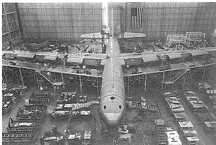
By May 1948, the XB-36 was taking final shape in the experimental building. (Photo—Convair). At right, the engine test stand outside the experimental building on which hundreds of test hours were run. (Photo—Convair, courtesy of Dalton Suggs)
