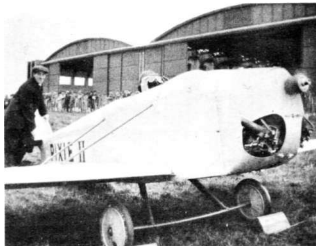
The Parnail "PIXIE II" was flown by Courtney a number of times at lightplane competitions. He is shown here and below in the cockpit, with goggles as the only windshield. Above photograph taken at Lympne, 1925. The engine was a Blackburn motorcycle engine,
