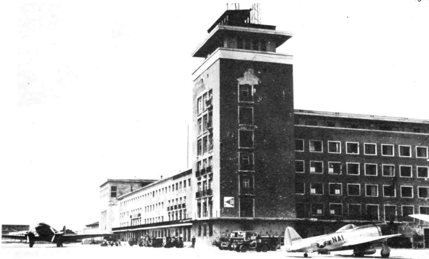
The control tower at Rheim, with rebuilt sections and fragment damage still evident. Col. Edwinson's NA-1 at the right.
