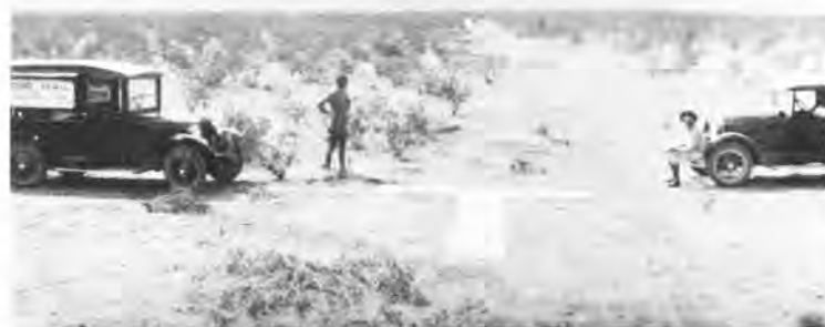
Remelin and DeGarmo laying out the landing "T," somewhere on the desert along the route from Los Angeles to Salt Lake City, February 1926. The canvas markers indicated emergency strips approximately every 20 miles.
