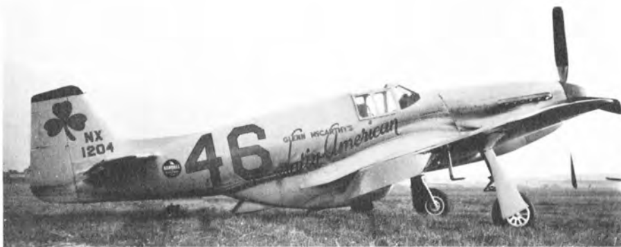
Figure 4. Paul Mantz entry in the 1948 Bendix. Aircraft is a P-51C-10-NT (AAF 42-103831) modified to incorporate a "wet wing" for long range nonstop transcontinental flying. (Photo — Charles Mandrake collection)
